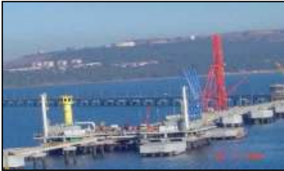
Figure 14. BTC pipeline jetty.
