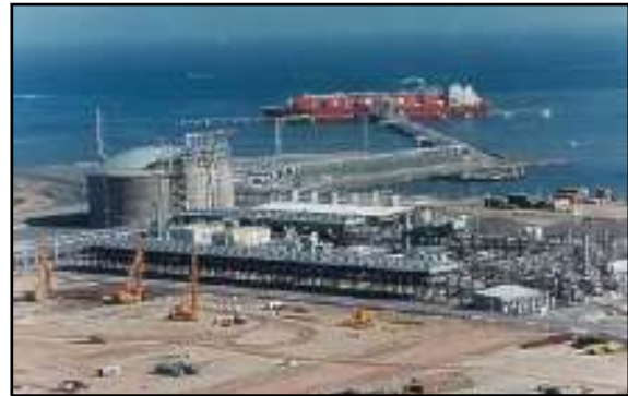
Figure 8. LNG terminal with tanker unloading.
